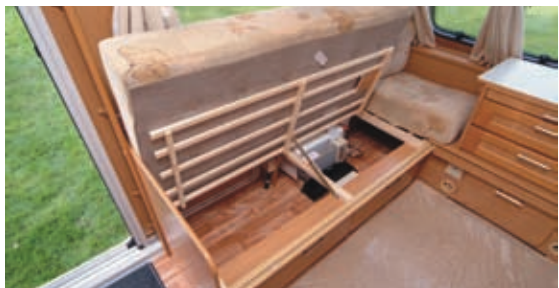
The fuses and cut-off switches at the front of the bed box impede access
